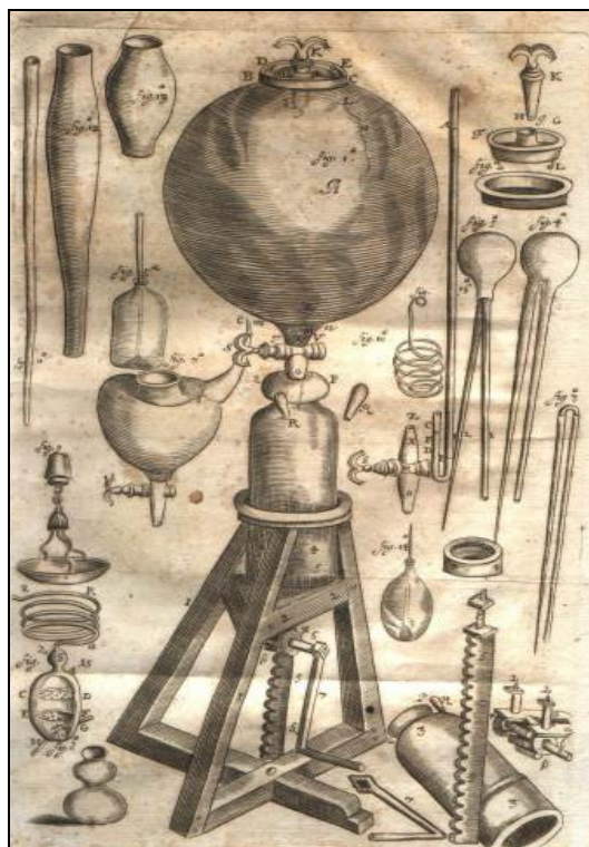
Fig. 4. The air pump constructed by Robert Hooke and Robert Boyle (1667)
